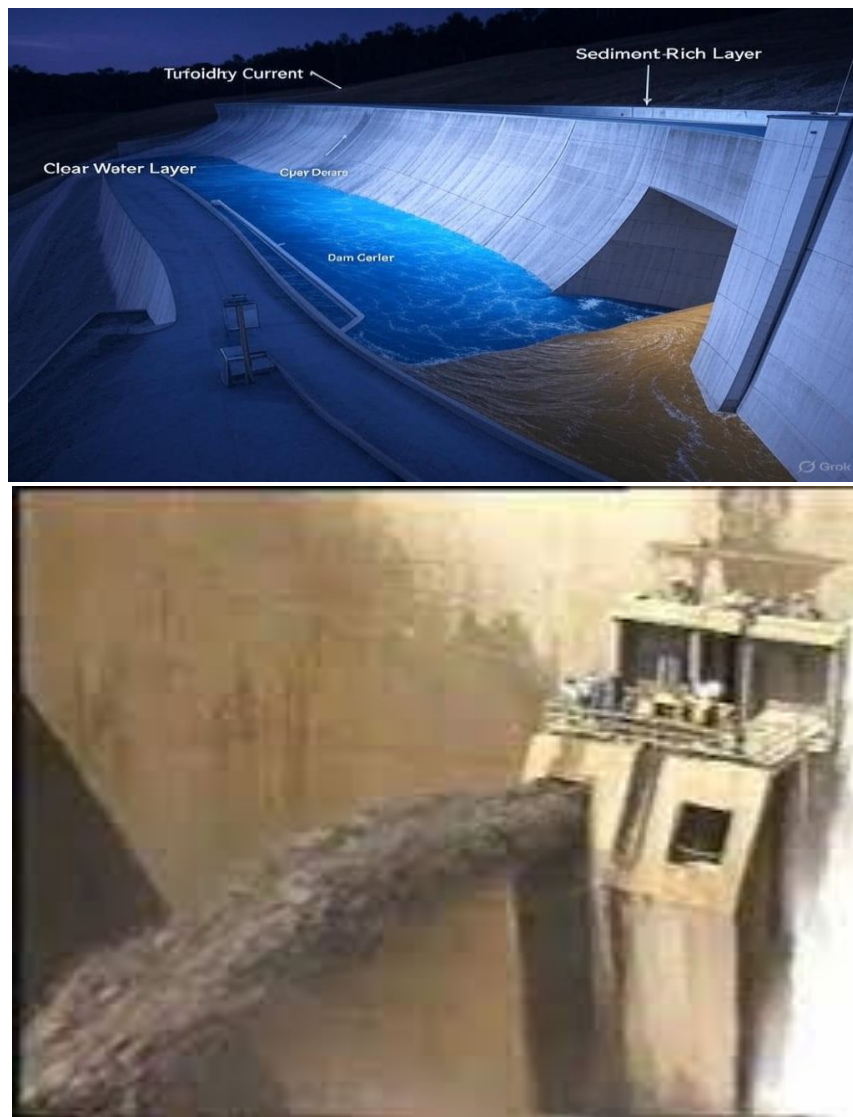
Figure (4) the successful hydraulic flushing through Gravity Concrete Dam
