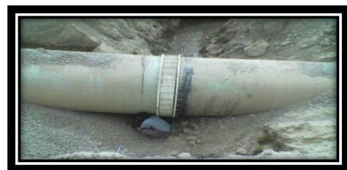
Figure (9): There is erosion under the GRP pipe bed Image
