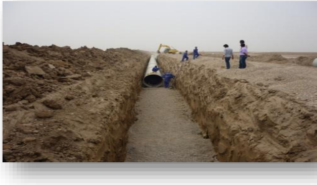
Figure (6) A view of GRP piping in vertical trench with appropriate substrate
