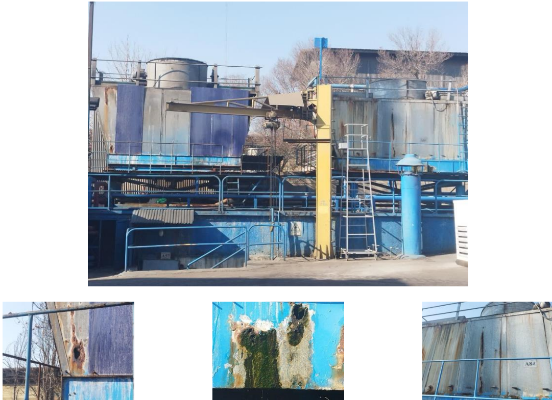
Fig. 6 Current damages observed in the open-circuit evaporative cooling tower
