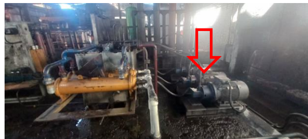
Fig. 5 Cooling hydraulic pack oil pumps to increase the lifespan and improve the efficiency of the pumps
