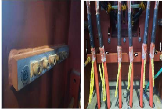
Figure 2: Corrosion in the electric motor power panels.
