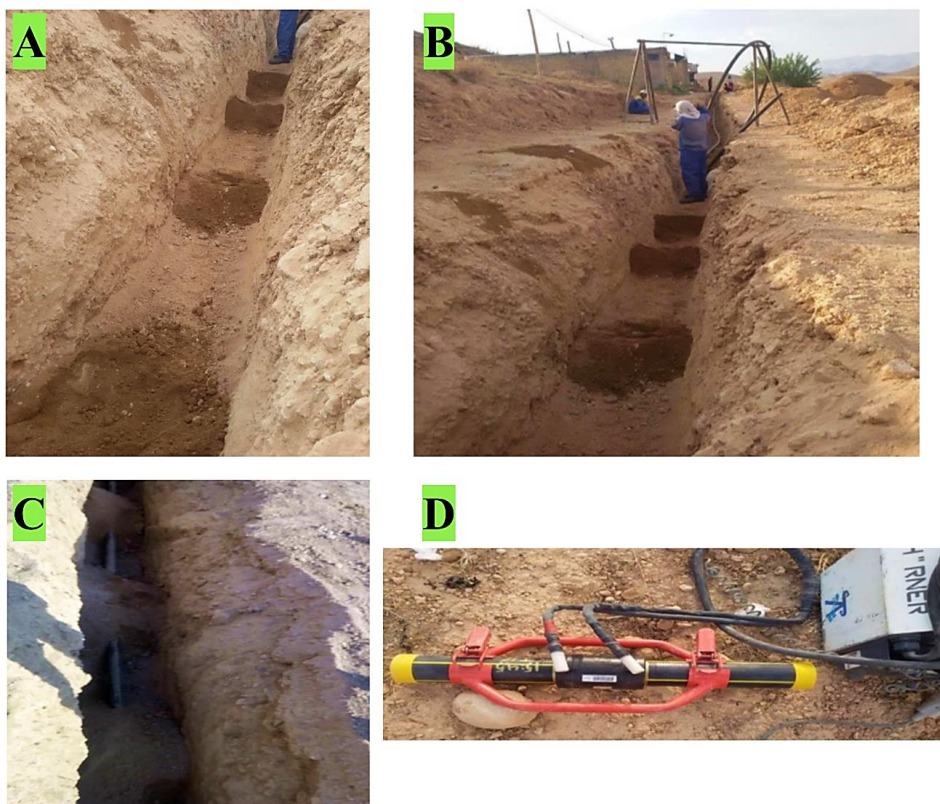
Fig. 1 Cushions created in the channel (A), how to place the pipe in the channel (B), covering the tube on the Cushions after tube placement (C), electrofusion welding in open space - gas delivery (D)
