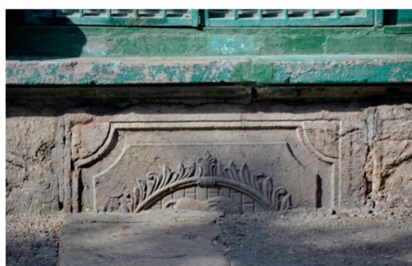
Figure 20- The external stone plinths of the building consist of five pieces of carved stone, part of which is hidden in the covering of the current passage (Archive of Tehran City Beautification Organization)
