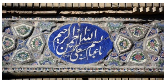
Figure 14- The tile inscription of the date of the building and the name of the founder "Abbas Ali" on the front of the building in 1895, the details of the tile work around it with enamel glaze and in relief (Tehran City Beautification Organization Archive)
