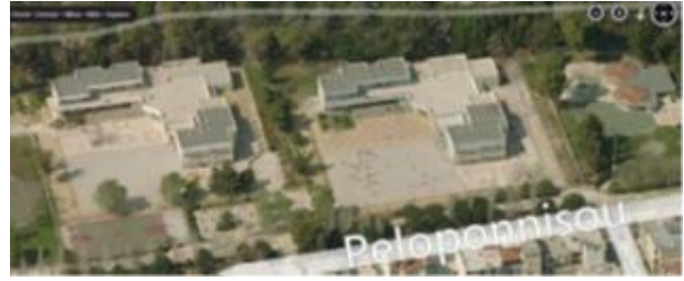
Figure 4: reference building and tested building
