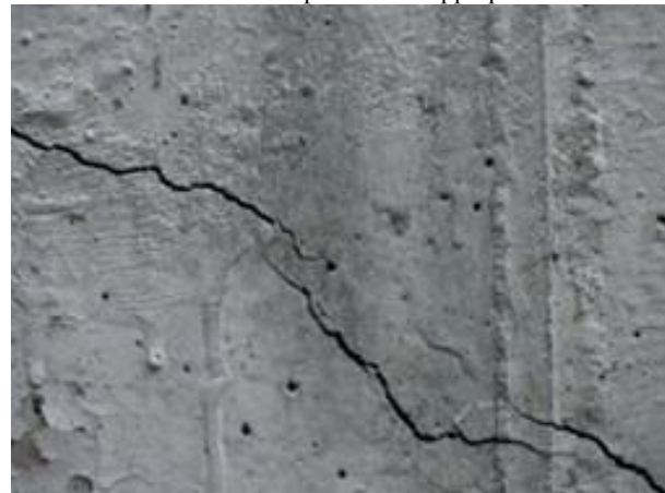
Figure 2. View of concrete surface
