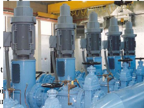
Figure 2. A vertical pumping station using shaft and sheath pumps.
