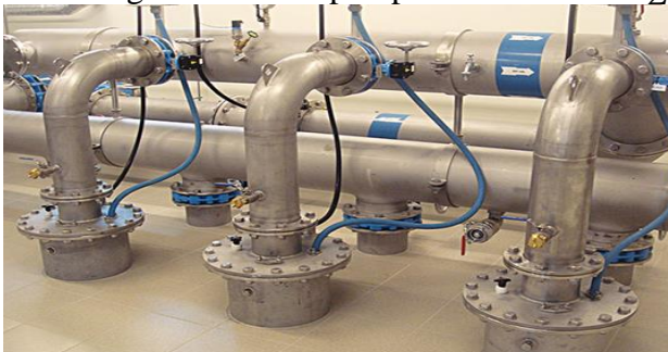
Figure 3. Vertical pumping station using floating pumps.
