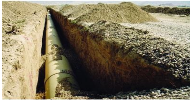
Fig 9. Execution of the GRP pipeline
