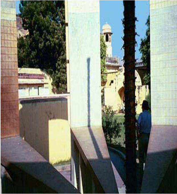
Fig. 17. With sunrise, indicator shadows moves on graduated planes. (Source: Daulat Singh Rajawat)
