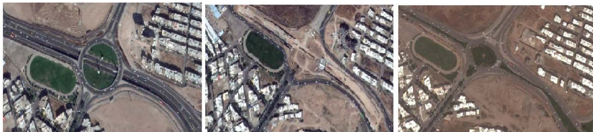
Fig. 3. Aerial photo of Nasr overpass in three construction phases: Before the construction, during the construction, after the construction
