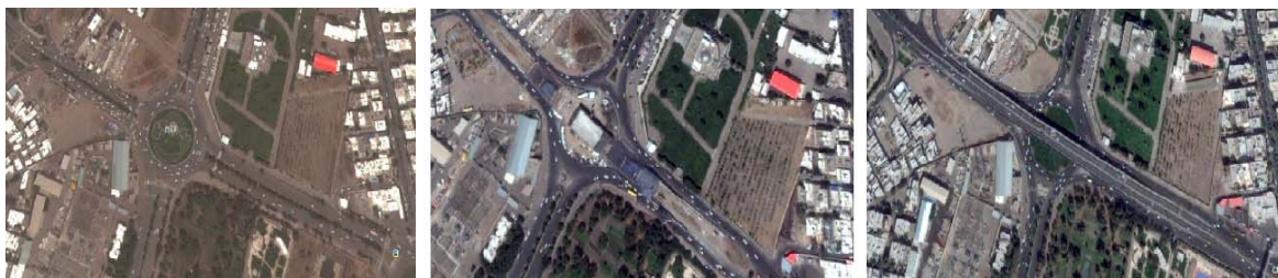
Fig. 4. Aerial photos of Sardaran overpass bridge before the construction, during the construction, after the construction.
