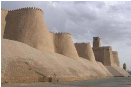
Fig. 23. View of the western walls including those of Kuhna Ark (Piperno, 2017:1)
