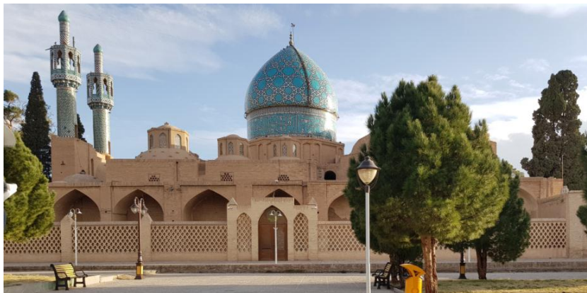
Fig. 13. Image of the northern front of the Astaneh where the dome and the two minarets of the Vakil al-Mulki courtyard can be seen.
