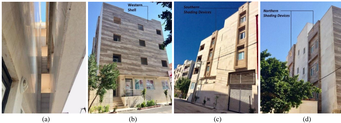
Fig. 6. a) The void behind the western shell, b) western shell, c) south facade, and d) north façade
