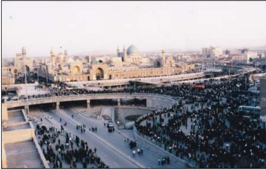
Fig.9: The underground circular road around the holy shrine.
