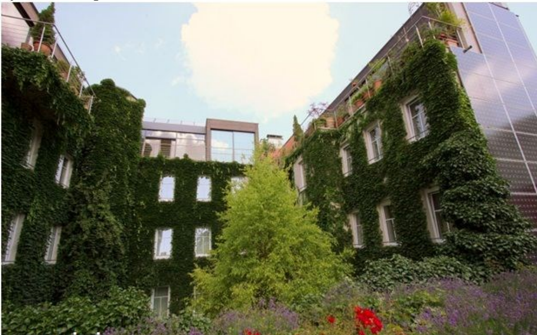
Figure 1 .Stadthaus boutique hotel, the world's first green hotel in Vienna, Austria
