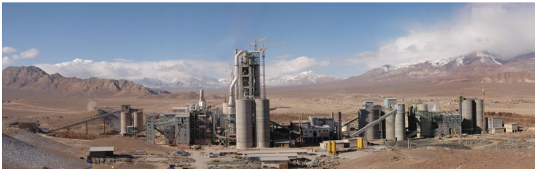
Fig 2. Shahrood cement plant.
