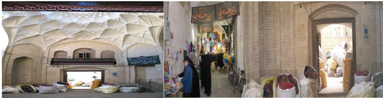
Fig.7. Mirafzali commercial building
