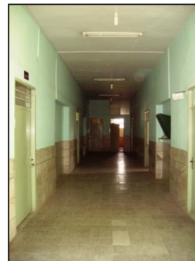
Fig.12: Corridor of ground floor of Shahrivar 17th School
