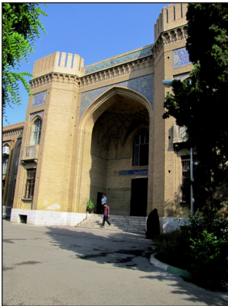
Fig.13: Entrance yard of Alborz School
