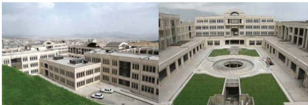
Fig. 3 and 4: Islamic Republic Academies by Naghsh consulting engineers (Source: http://www.maskanshahrsazi.ir )
