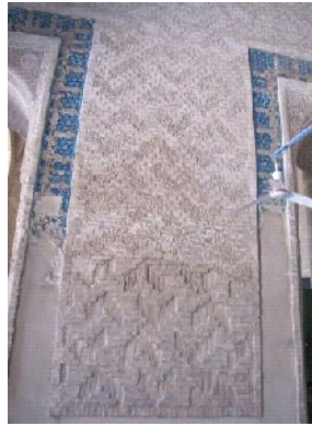
Fig 30 . 3: Break work cover on the structure in the dome chamber
