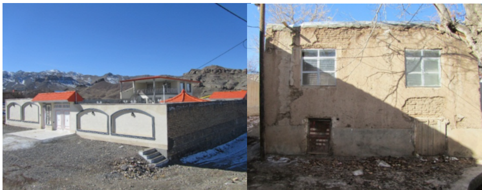
Figure 6: Renovated and hollowed units in Veshnaveh village
