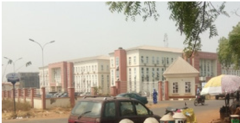
Fig. 7: Approach gate to the secretariat building
