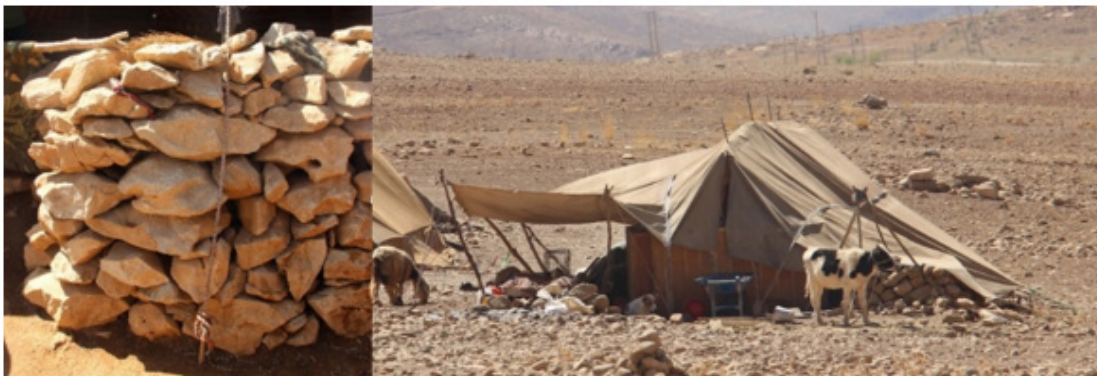
Fig. 19. Arrangement of the stones without mortar.
