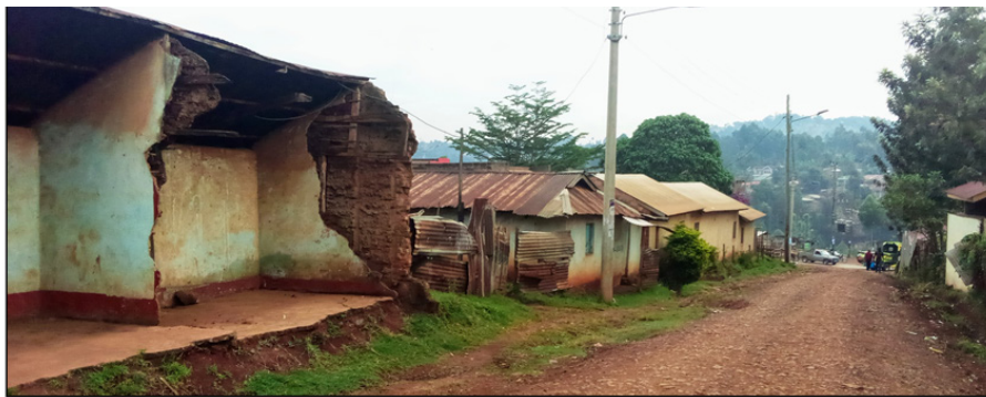
Fig. 6: A residential building demolished in Daraja Mbili for illegally being on a road reserve
