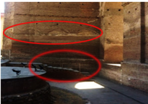
Fig. 11: Stairs leading to the basement of Ali shah's tomb
