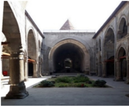
Fig. 17: Existence of a columnar vaulted courtyard in the building of two minarets of Erzurum
