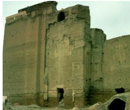
Fig. 4: Exterior view of the western wall
