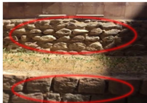
Fig. 12: Evidence of the use of rubble and cut stones in the basement of the building
