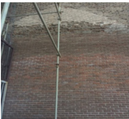
Fig.13: Arches above the right wall
