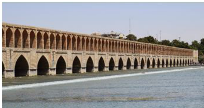
Fig.1: Allahverdi khan bridge
