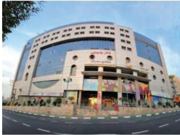
Fig. 3: Image of the Samarkand Commercial Complex in Tehran
