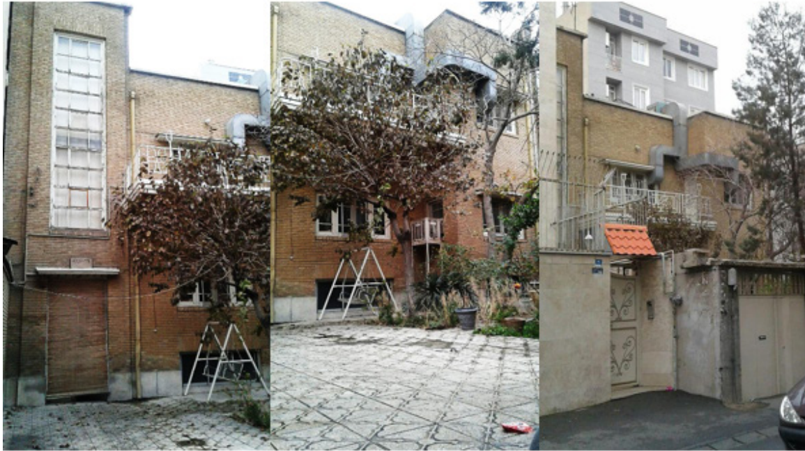
Fig. 6: The facade of a residential building in the Moniriyeh region, Tehran.
