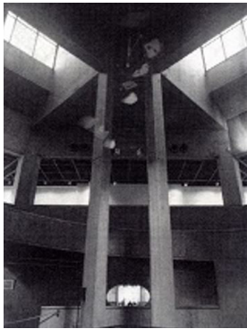
Fig. 16: Museum of Contemporary Art, Tehran, The exposed concrete columns of the interior
