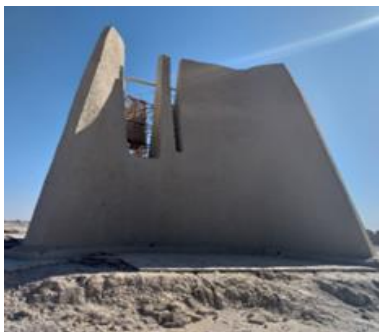
Fig. 15. The actual vault specimen located on-site
