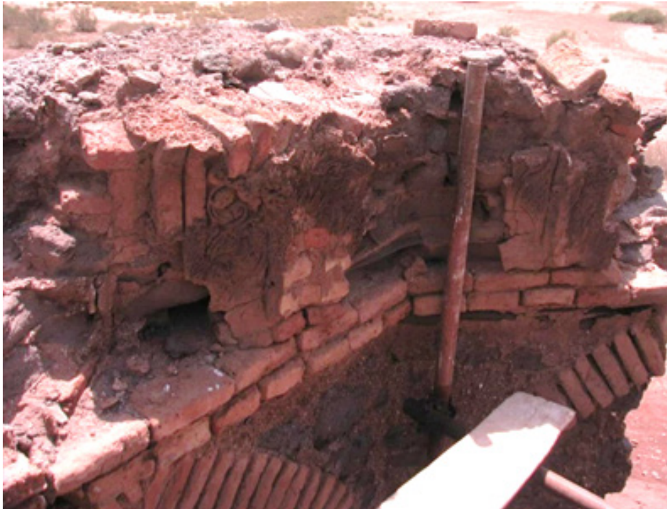
Figure 6: The brick support structure in the dome's shaft
