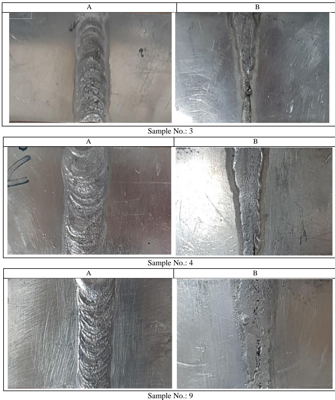
Figure 3. A and B show the top surface and the root of the weld appearance in the confirmed parts after the VT
