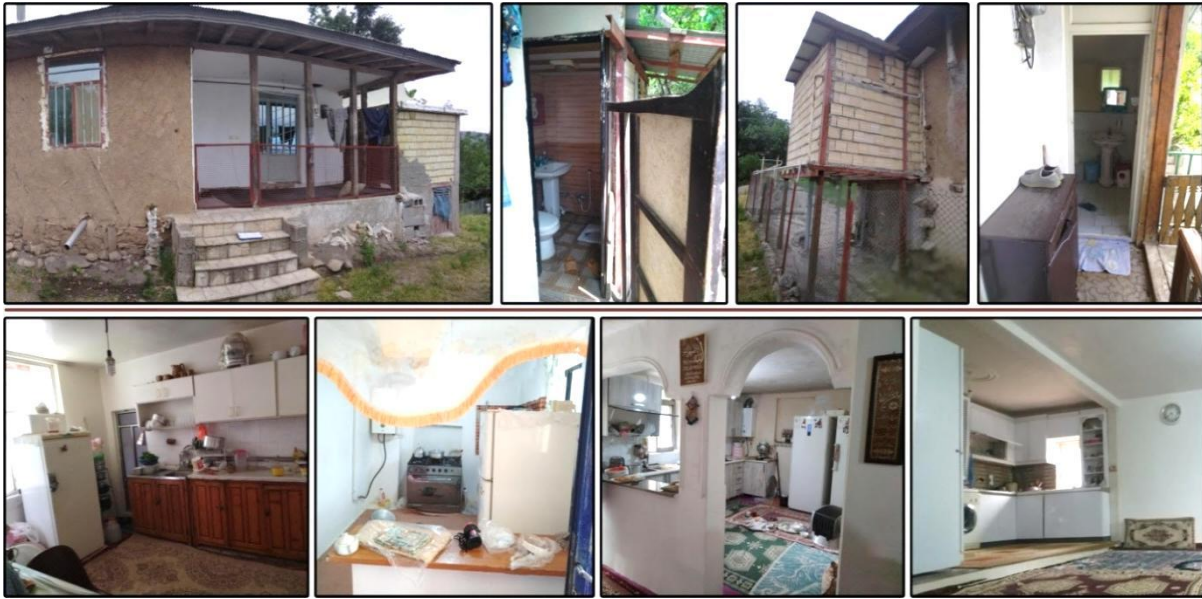
Fig. 6. Moving the toilet from the courtyard to the veranda (top pictures) and creating a separate kitchen (bottom pictures).
