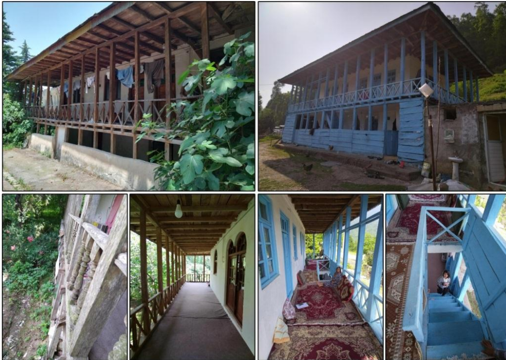
Fig. 3. Houses in Divarash (left) and Shirkooh (right) that were completely intact in the earthquake.
