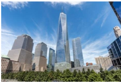
Fig. 2. One World Trade Center (New York City, USA), Completed in 2014.
