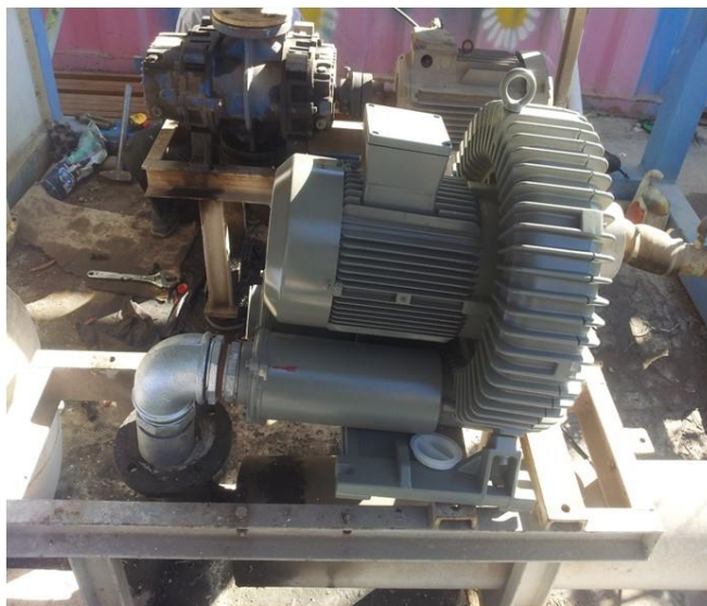
Helicoidal blower in the system under study (After the change)
