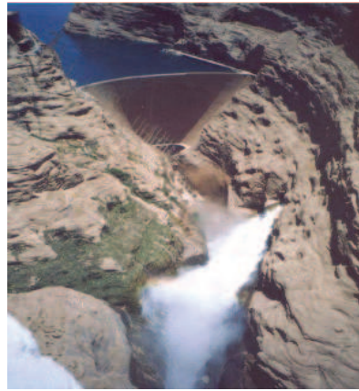
Fig.1: General view of double curvature arch of dez dam of Dez
