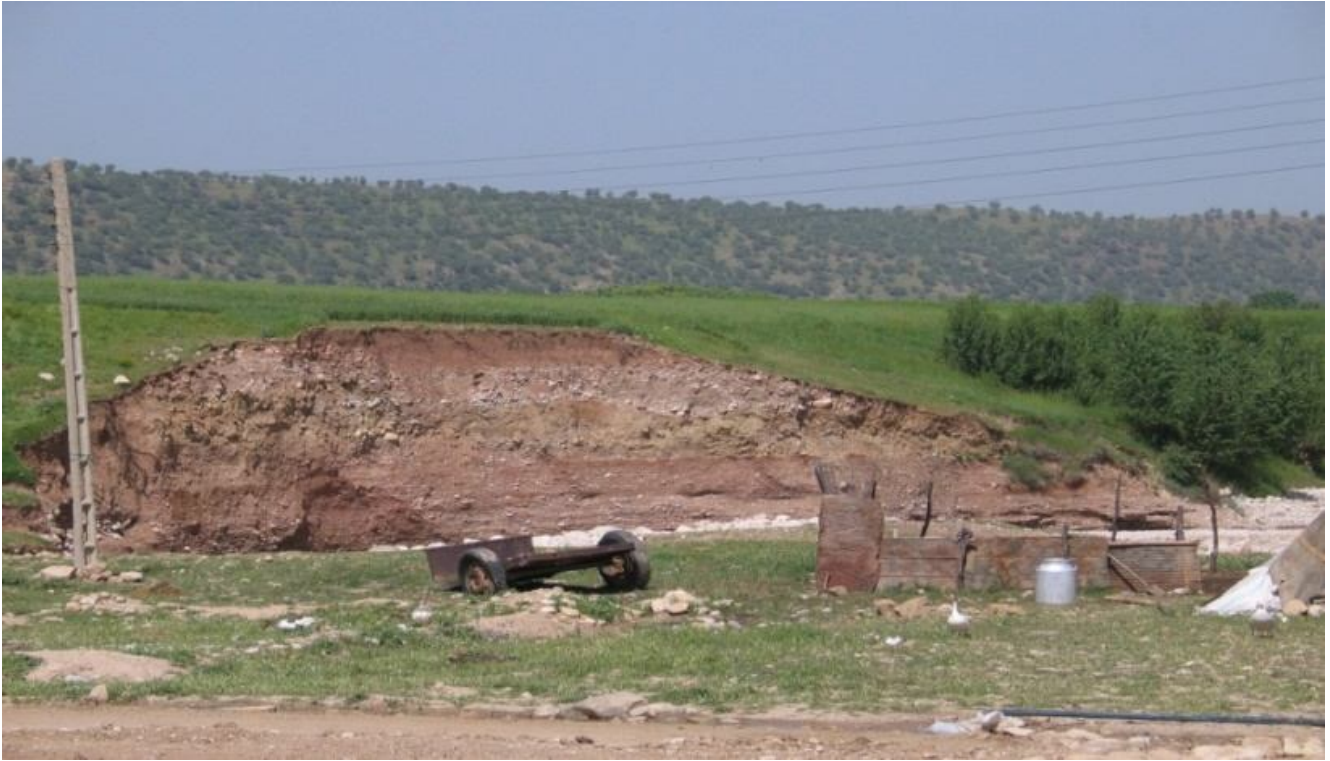
Figure 3. Occurrence of landslides due to river activity in the study area
