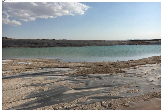
Figure 2. The view of the Kaveh industrial effluents transmission channel
