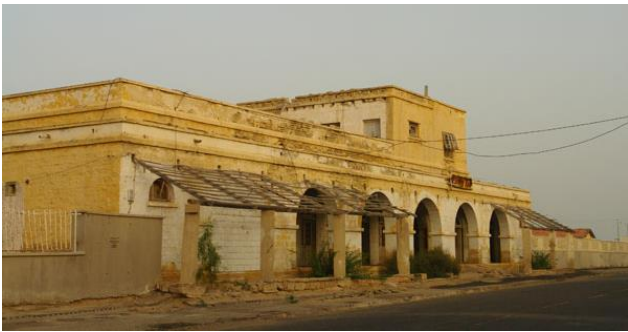
Figure 26. Old building Telegraph
