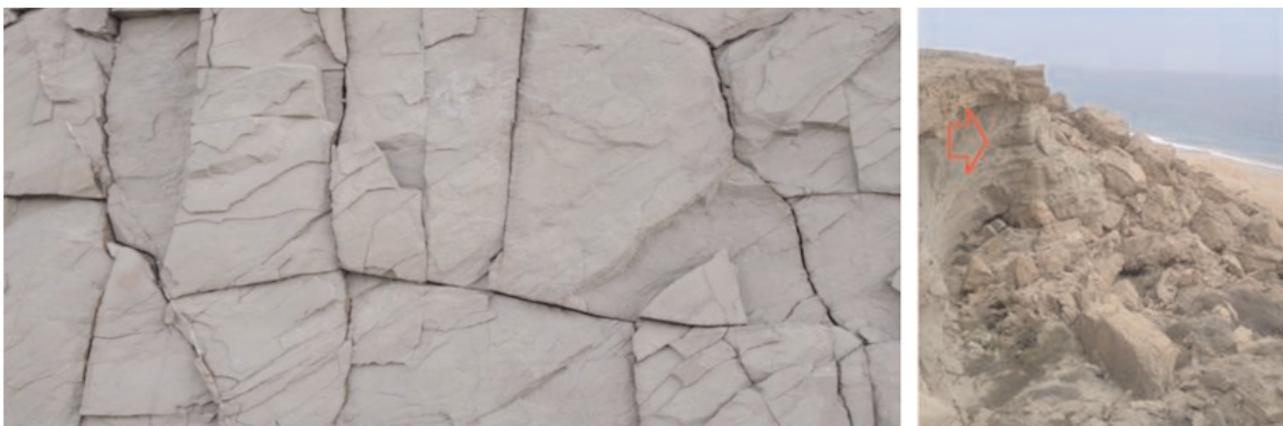
Figure 18. Fractures, slump and landslide in Makran coasts
