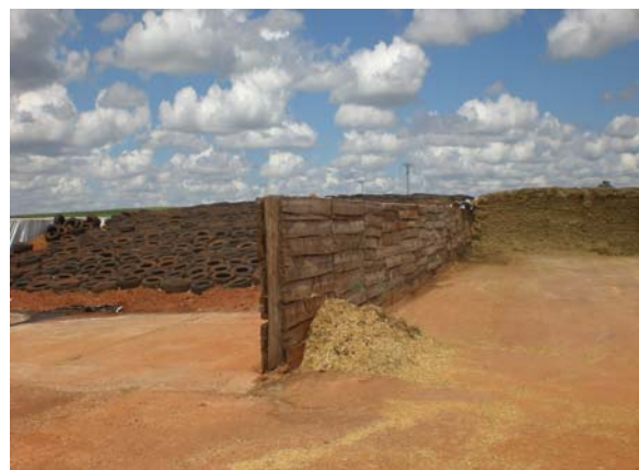
Figure 2 A silo divided by a wall in the middle to avoid aerobic spoilage under Brazilian practical conditions
